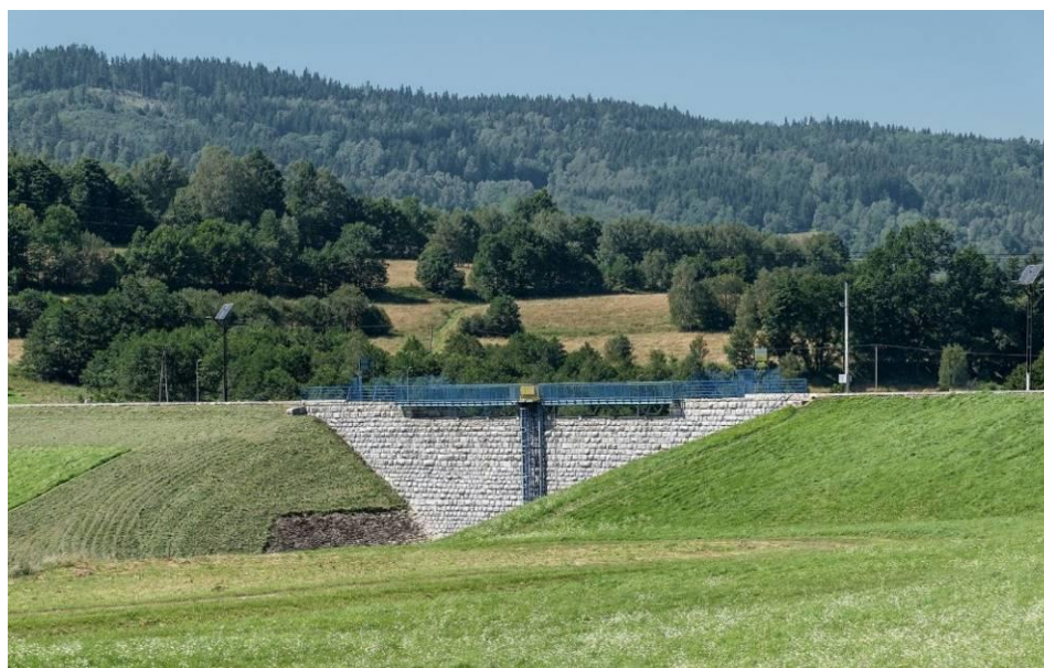
Figure: 43. Detention pond (source:
