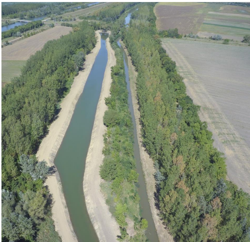
Drone photo of the executed storage area
